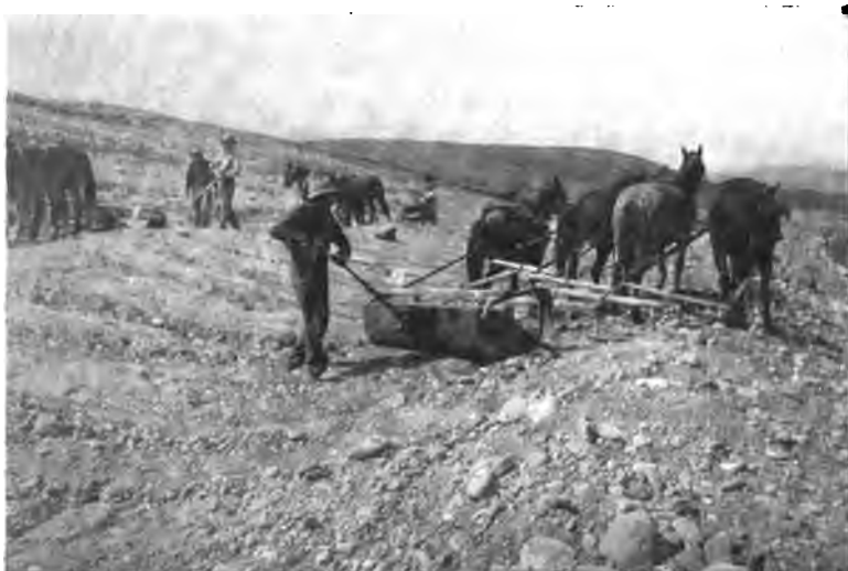
FIG. 77.—Building Canal with Fresno Scrapers.
